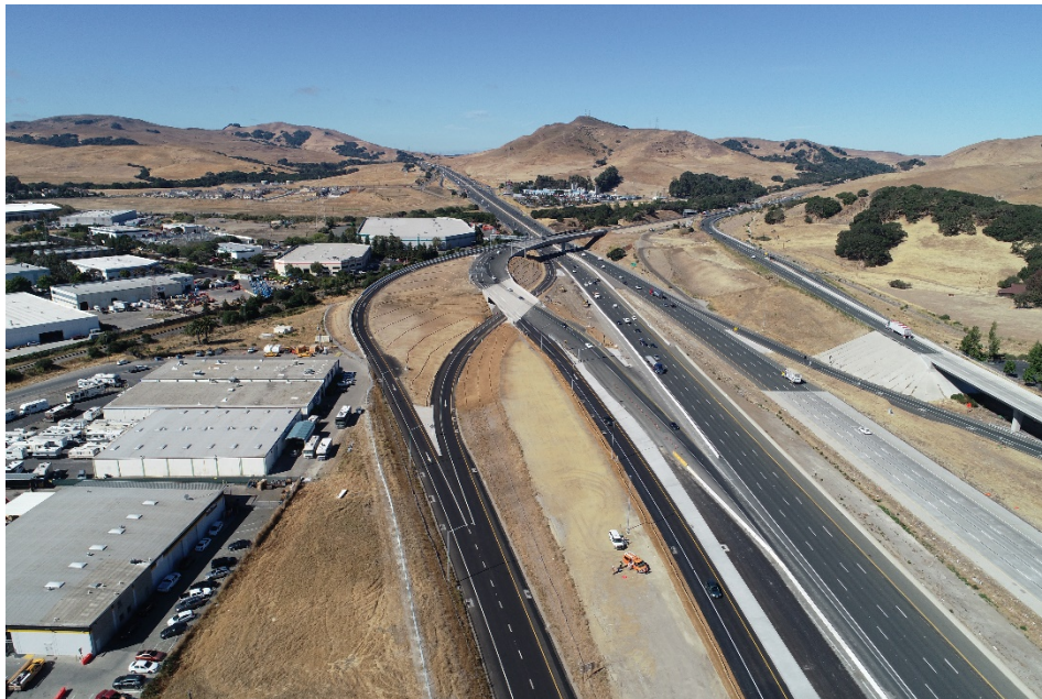
Aerial view of the newly-constructed I-80/I-680/SR-12 interchange in Fairfield
