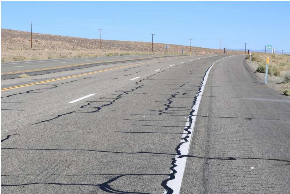
Before Picture of U.S. 395 in Inyo County
