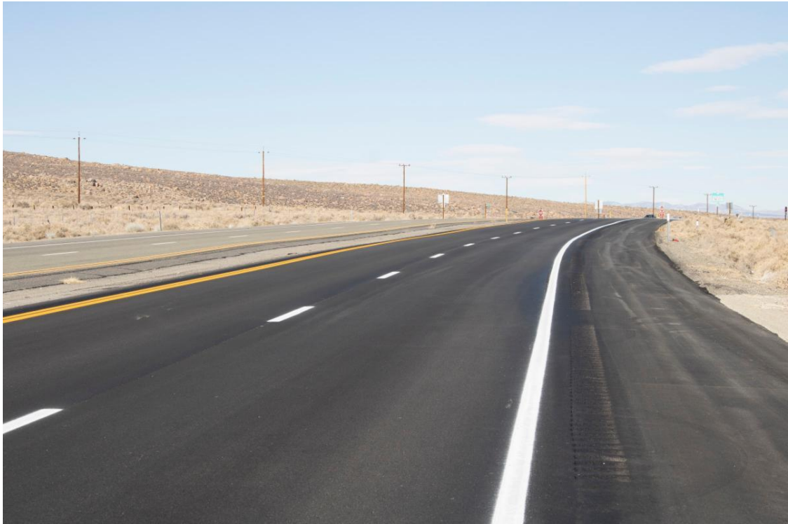
After Picture of U.S. 395 in Inyo County
